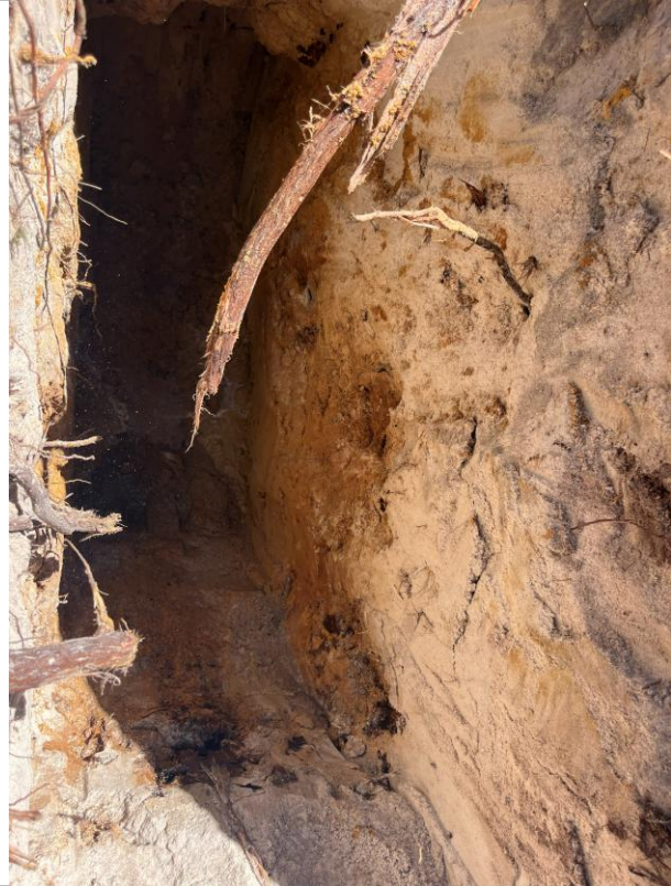
Development of Test Pit 3 (TP3)
