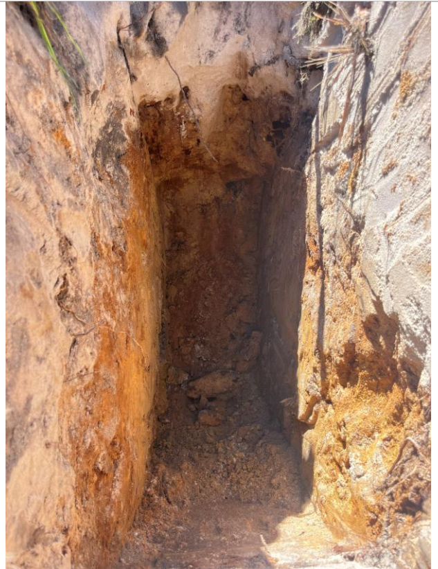
Development of Test Pit 2 (TP2)
