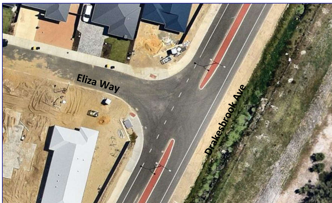
Figure 3.3: Drakesbrook Ave and Eliza Way Intersection (Streetview Sept 2025)
