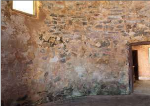
Image 35: Internal rough coarse limestone walls
