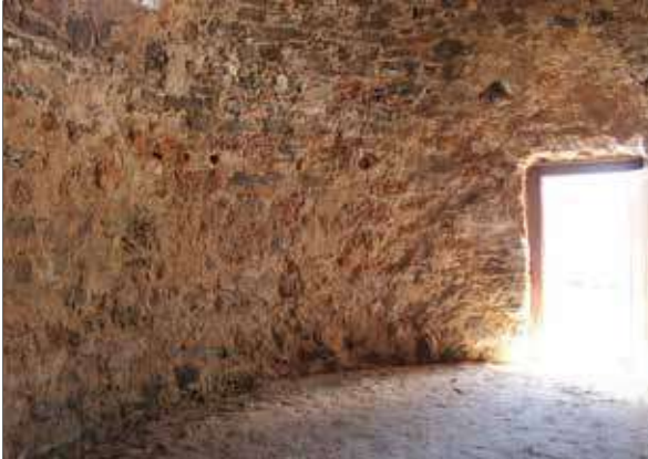
Image 33: Internal rough coarse limestone walls
