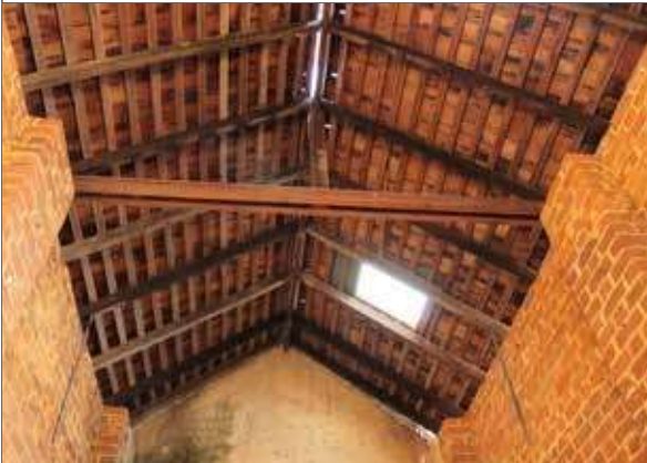
Image 41: Roof structures and skylight
