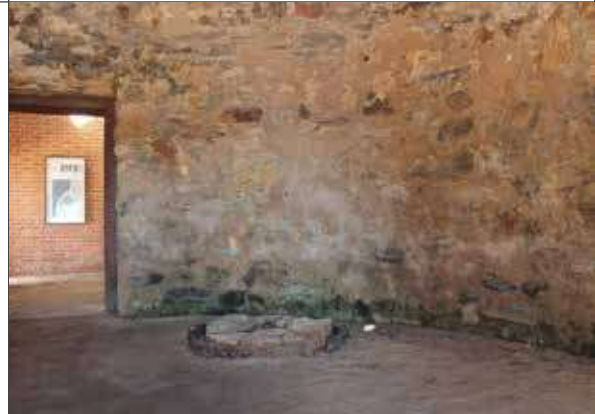
Image 36: Door to Engine Room
