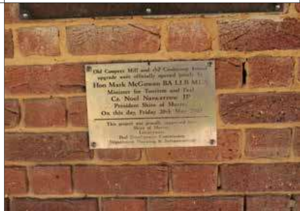
Image 32: Steel plaque to south elevation
