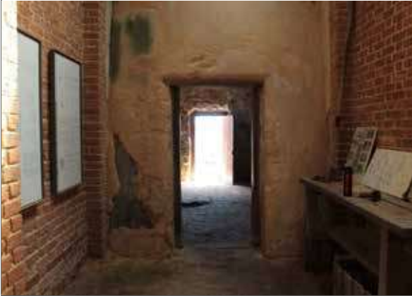
Image 39: Opening to mill
