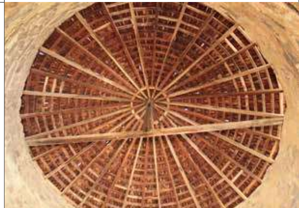
Image 38: Timber roof structure
