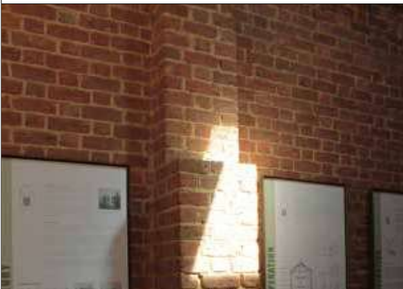
Image 43: Brick stepped engaged piers
