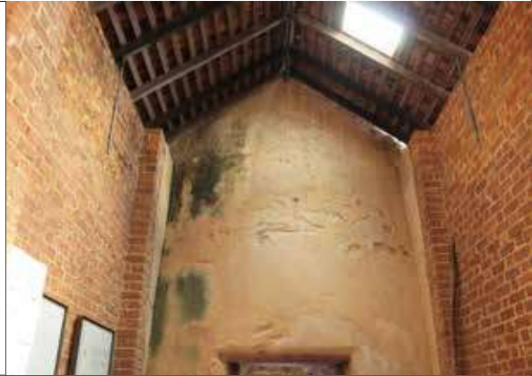
Image 40: North wall to Engine Room
