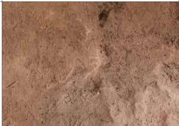
Image 44: Silt build-up internally
