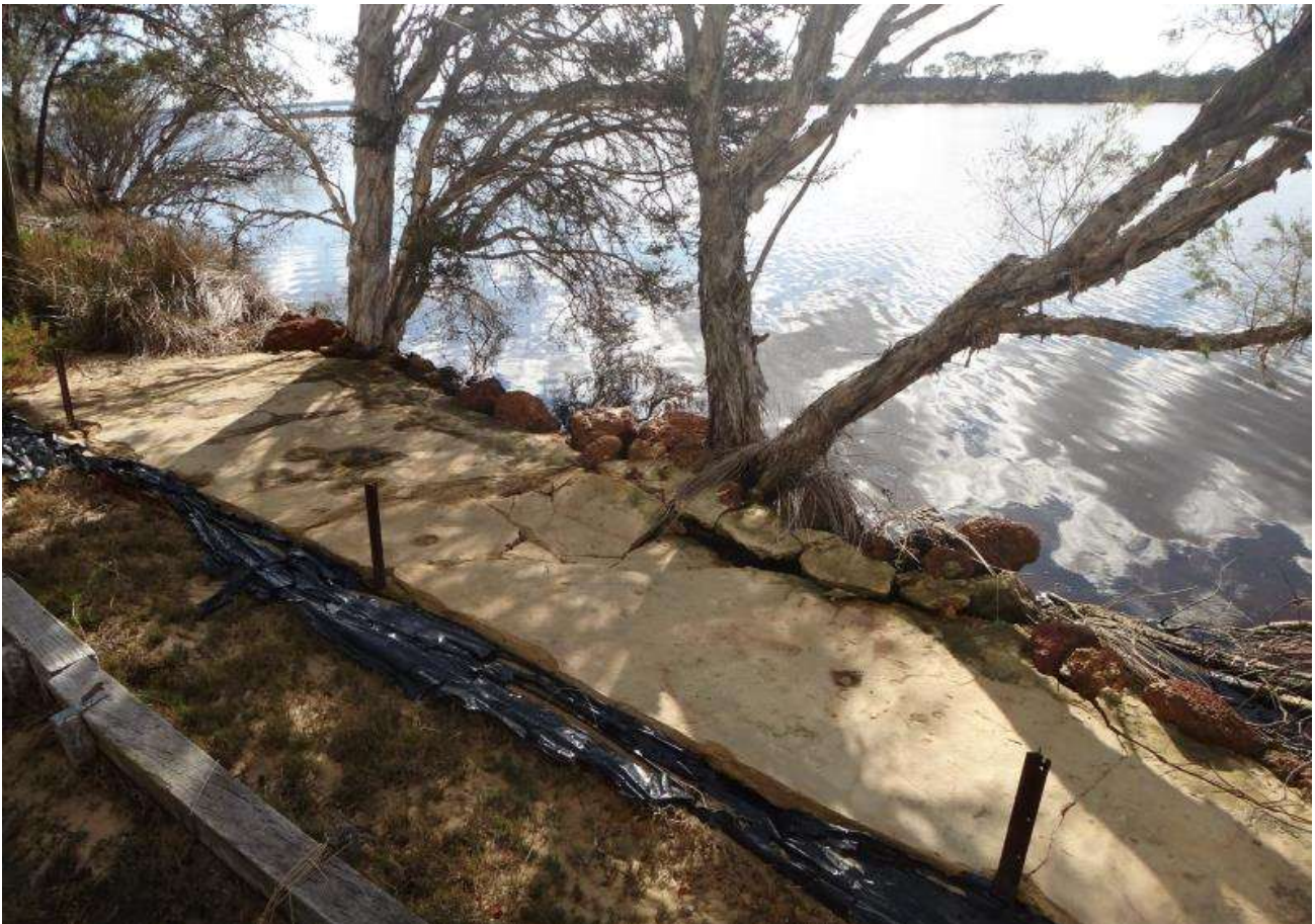
Figure 2-5 Winter 2011 – Northern revetment. New concrete capping installed. Supplied by Shire.
