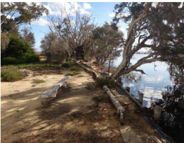
Figure 2-3 Winter 2011 – Northern revetment. Supplied by Shire.
