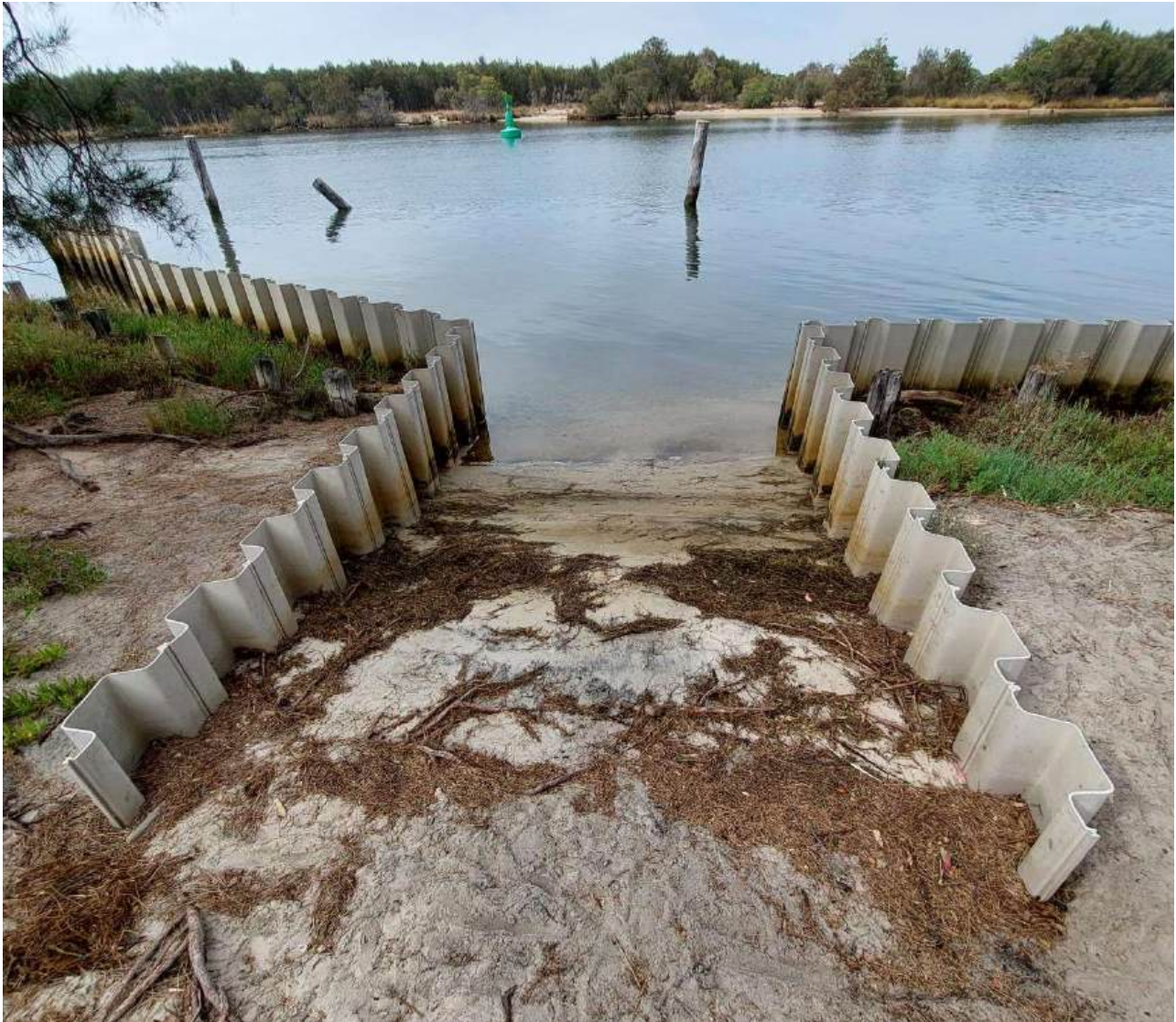
Figure 9-4 PVC sheet piled wall in place on the southern foreshore of the study area since ~2013.
