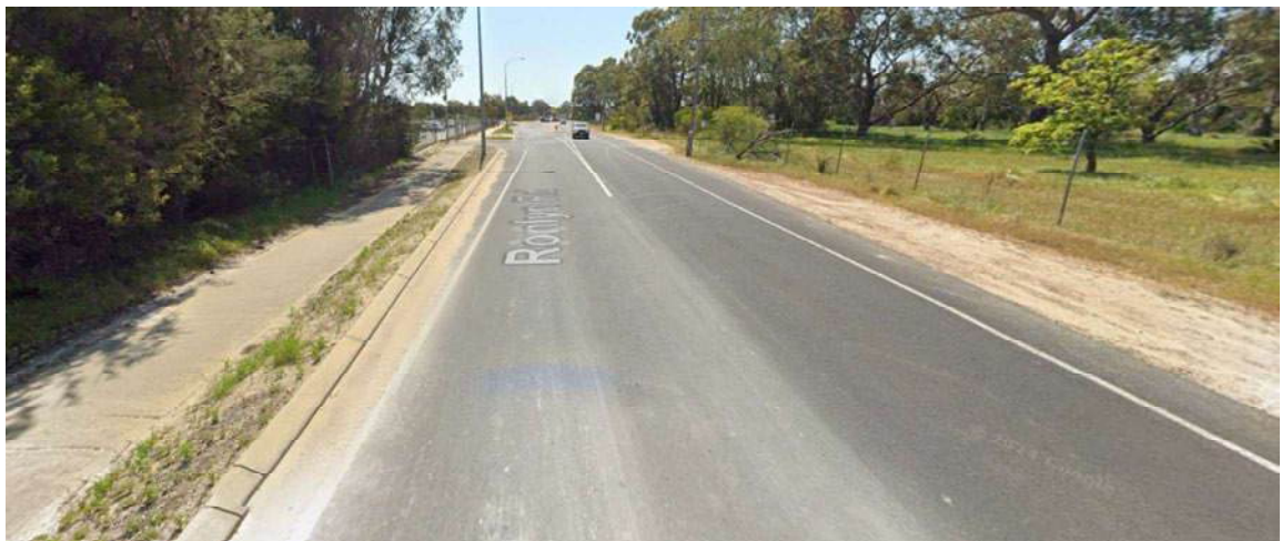
Figure 4: Ronlyn Road looking north in the vicinity of the subject site
