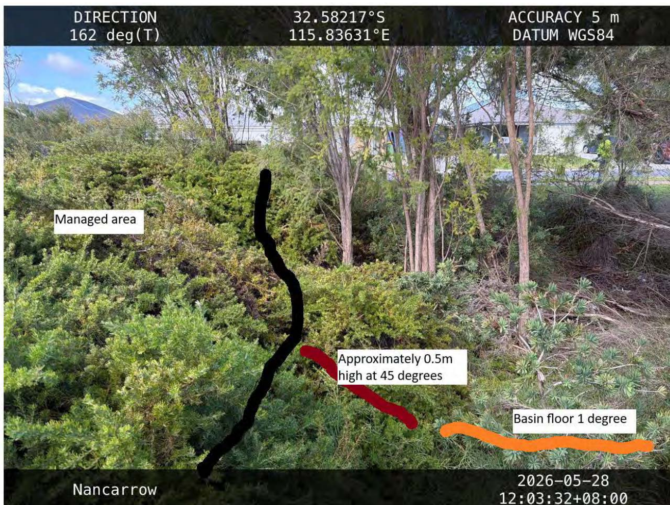
Photo detailing proposed managed area (black mark) between childcare site and basin, 0.5m 45 degree downslope from managed area to basin floor and basin floor.
