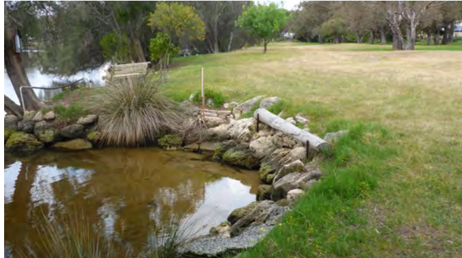
Low Bank Height, limestone rock revetment
