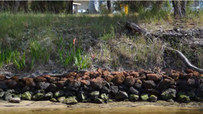
High Bank Height, rock armoured toe
