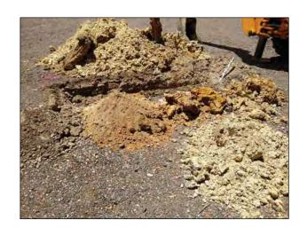
RIG: 8 tonne backhoe with 450 mm toothed bucket
