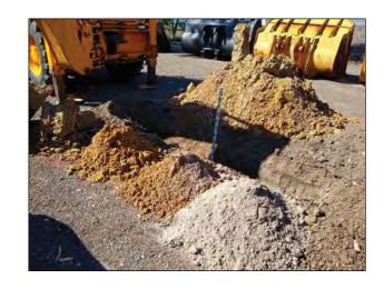
RIG: 8 tonne backhoe with 450 mm toothed bucket
