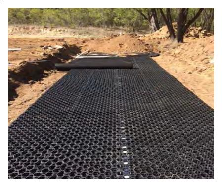
Plate 1: A flatbed leach drain being installed. Note the shallow depth of these which will maximise separation from groundwater and the impervious layer.
