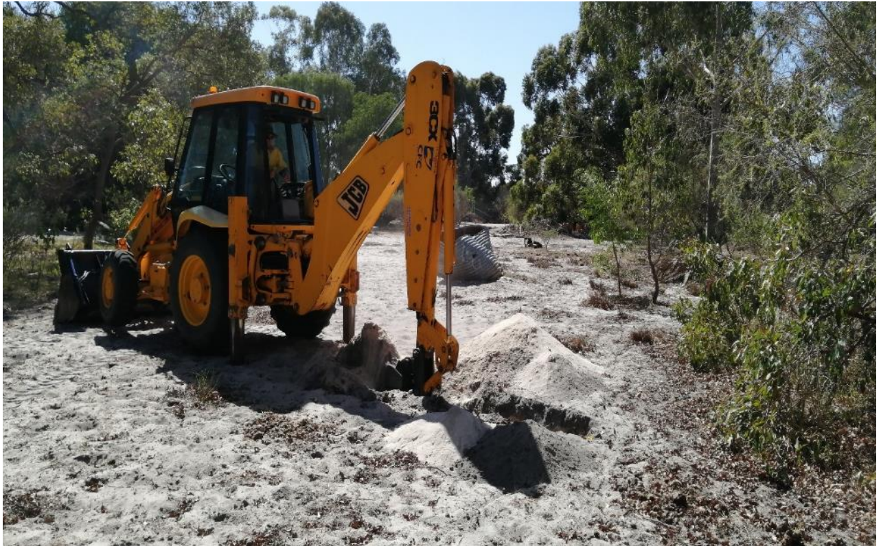
Photograph 1: Excavation of test pit at TP04
