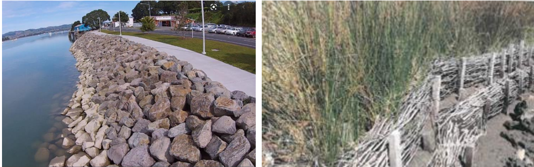
Figure 2-1. Example of "Hard" Engineering Solution (left) 3 and Nature Based Solution (right) 4
