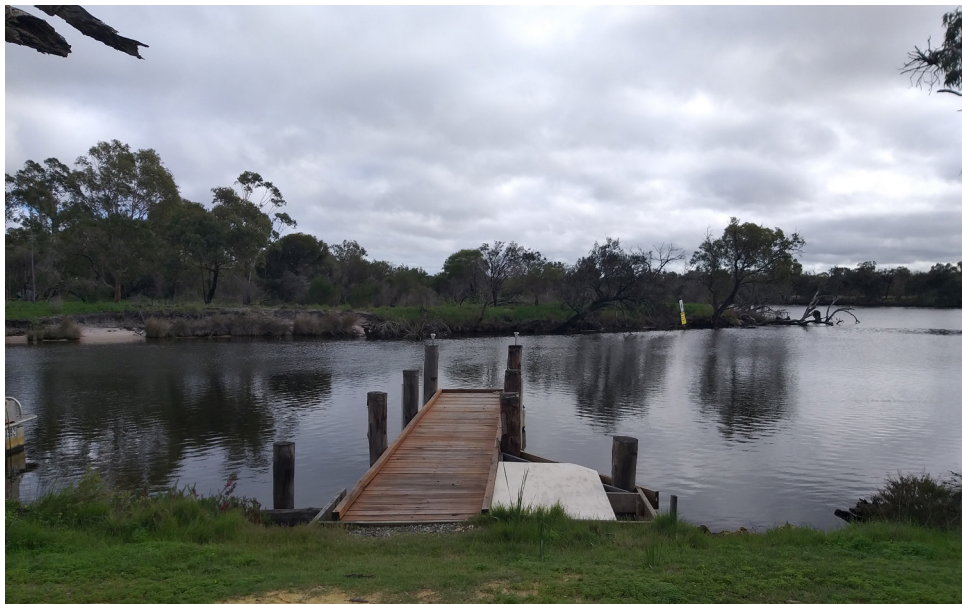
Flooding over jetty
