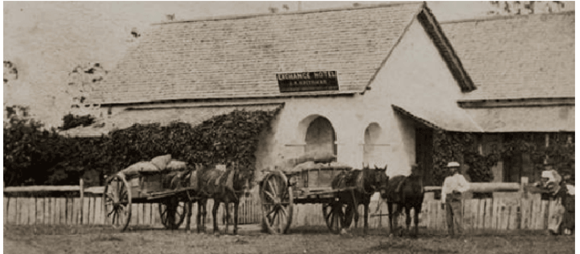
The earliest known photograph of the Exchange Hotel showing smooth rendered masonry with shingle roofing.
