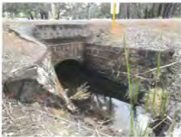
Figure 9: Curb at south end corner
