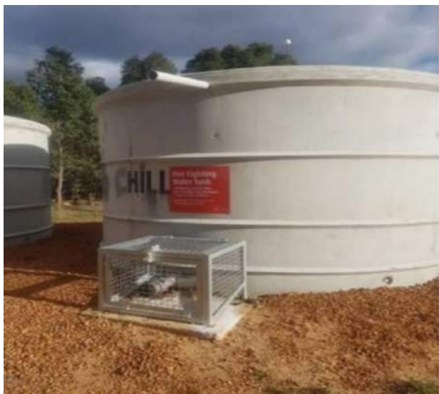
Strategic 47,000 Litre Concrete Tank & Protected Fittings
