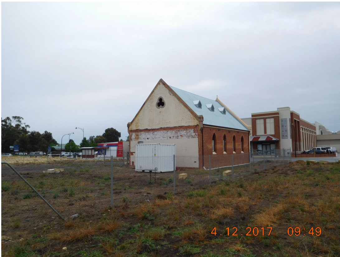
Photograph 04: View looking towards the south (rear) elevation of the Pinjarra Masonic Hall. Scars of former latter addition visible following removal. Griffiths Architects, December 2017.
