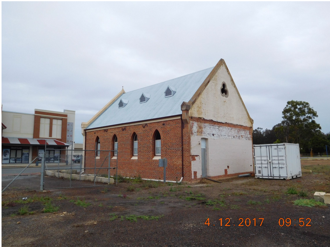
Photograph 05: View looking towards the south (rear) elevation of the Pinjarra Masonic Hall. Scars of former latter addition visible following removal. Griffiths Architects, December 2017.
