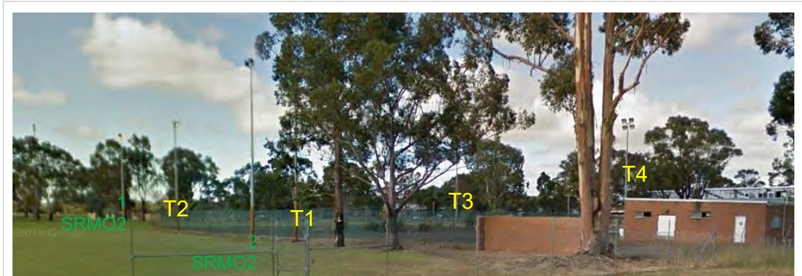
Sports lighting on Pinjarra Tennis Courts
