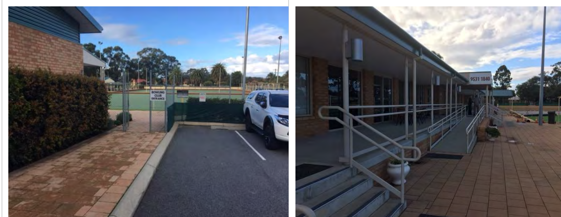
Bowling club entry from carpark
