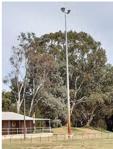
One of 3 existing floodlights
