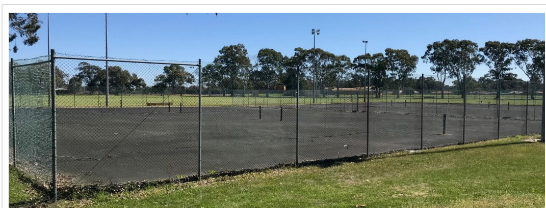
Pinjarra Tennis Courts - not in use
