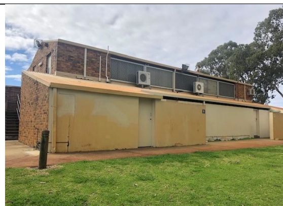
Rear view - facing the carpark
