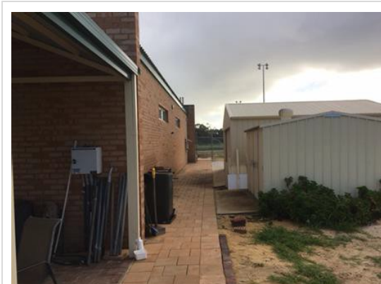
External storage to the north of the clubhouse
