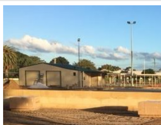
Main storage adjacent Green B
