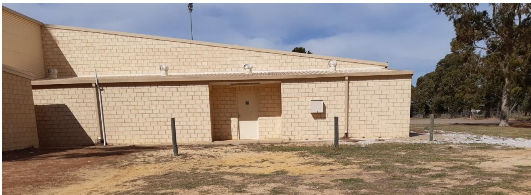
SRMO1 Public Toilets - entry to Male / Female / Disabled facilities
