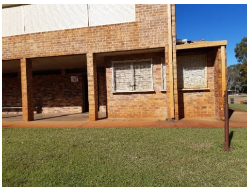
Kiosk servery on right
