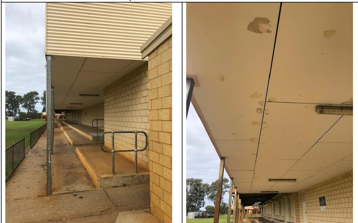
Viewing verandah west side of SRMO1
