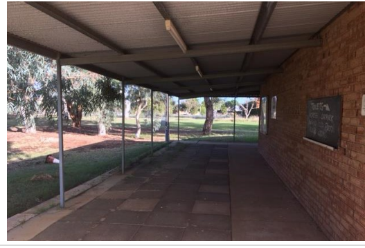
Verandah on east side of building
