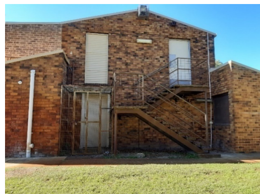
First floor egress and kiosk entry
