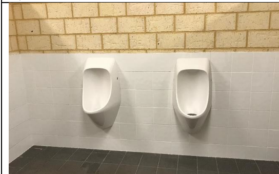
Urinals in the shower toilet area
