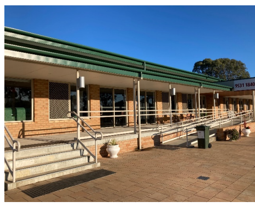
Bowling club entry from greens side
