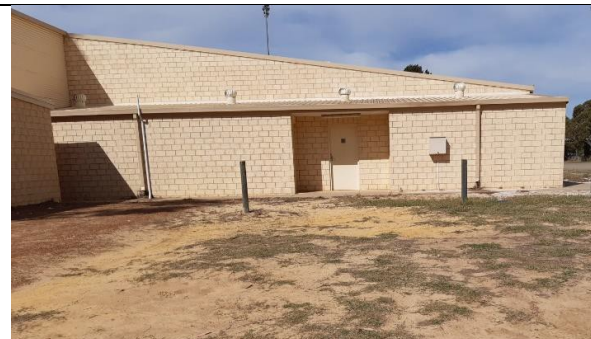
External public toilets - M / F / UAT
