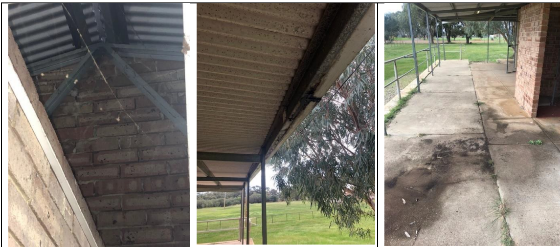
Roof is sound
